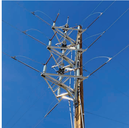
Remote motorized switches on a new transmission pole. This switch can feed the Florence, Waverly and Rauville substations from the north or south and open each substation for isolation.
