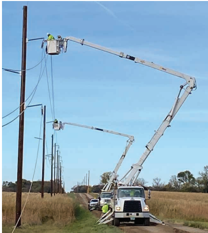
New line being strung on a line northwest of Henry.
