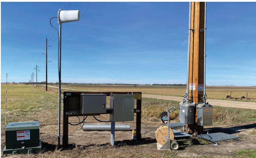
Controls for the motorized switch at the bottom of the pole.
