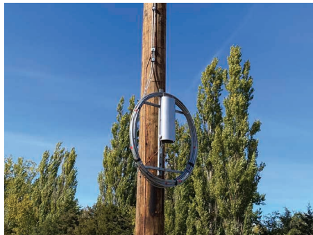
A spliced static/fiber cable in a coil. The fiber optics are spliced using a special tool. The splice itself is housed in the container shown.
