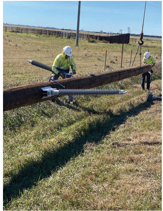
Insulators being bolted onto a new transmission pole
