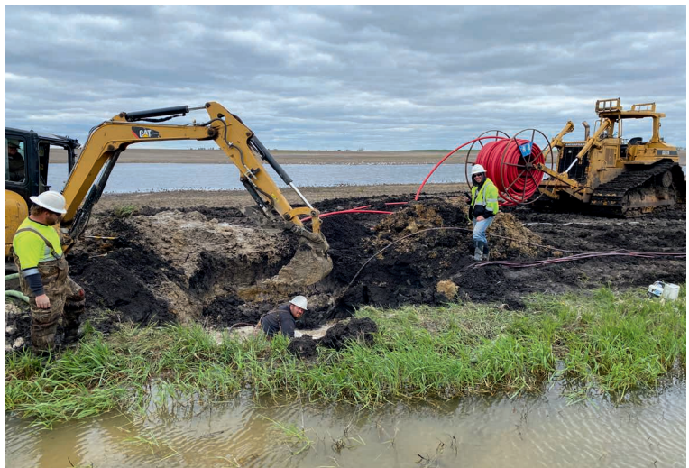
Shown at top is a boring machine on the south side of the road being bored. Shown above is the crew on the north side of the road using a trash pump to remove the water. They are working below standing water.
