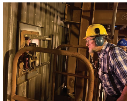
Marvin Hofer looks inside the 277-foot boiler at Antelope Valley Station.
