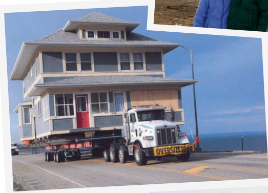
The house rounds one of the final corners. Southeastern Electric Cooperative was on the scene to connect power. Submitted Photo
