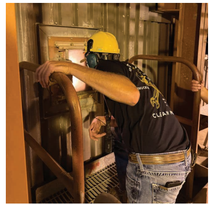
Dustin Beebe looks inside the 277-foot boiler at Antelope Valley Station.
