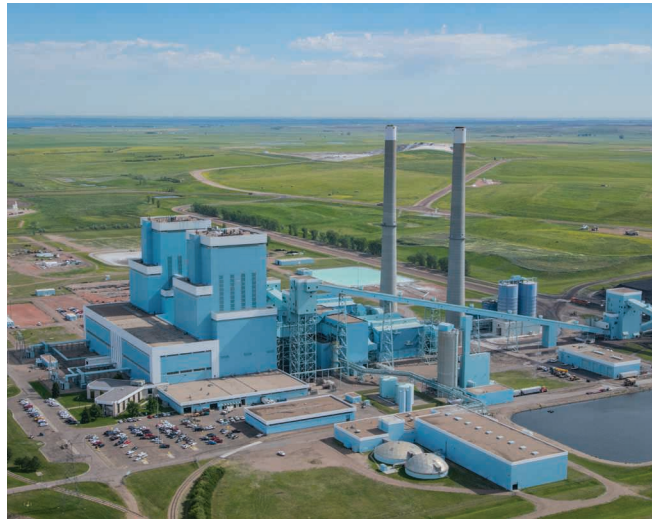
Antelope Valley Station power plant.
