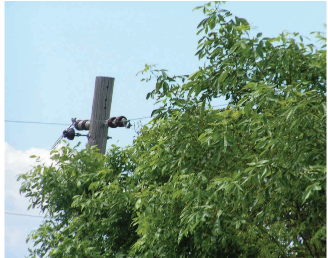
If you observe trees in the line as shown, please contact the Codington-Clark office with the location.
