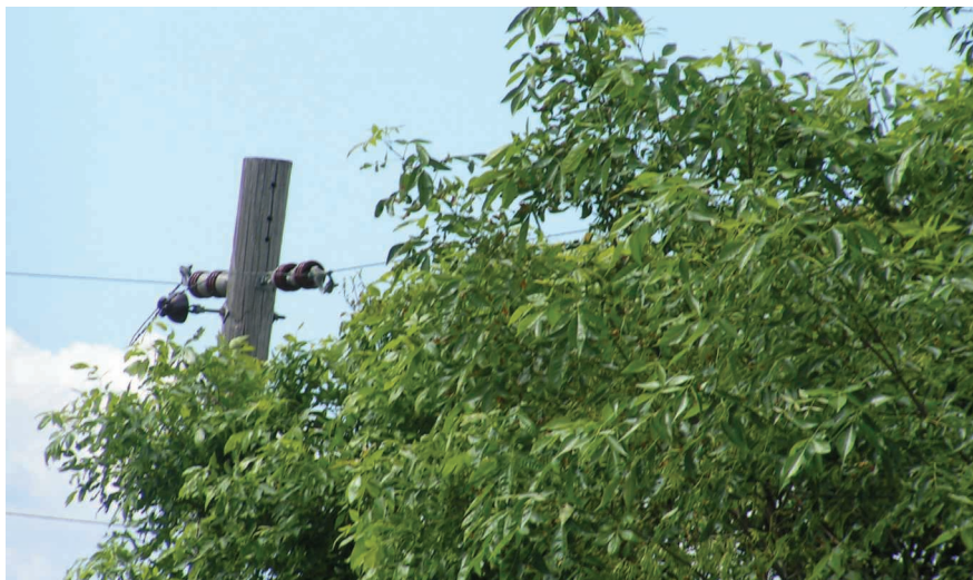
If you observe trees in the line as shown, please contact the office with the location.
